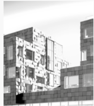
Exterior of Copenhagen International School, Nordhavn, designed by CF Møller (2017).
