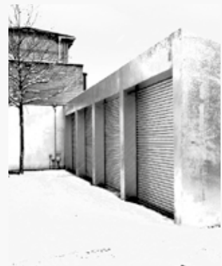
Artist’s studio, King’s Cross, London, designed by Carmody Groarke. The building is clad with galvanized steel.
