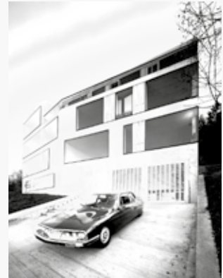
Architect’s and artist’s house, Zurich, Switzerland, designed by Andreas Fuhrmann Gabrielle Hächler Architects (2003). The building is entirely clad in galvanized steel plates.
