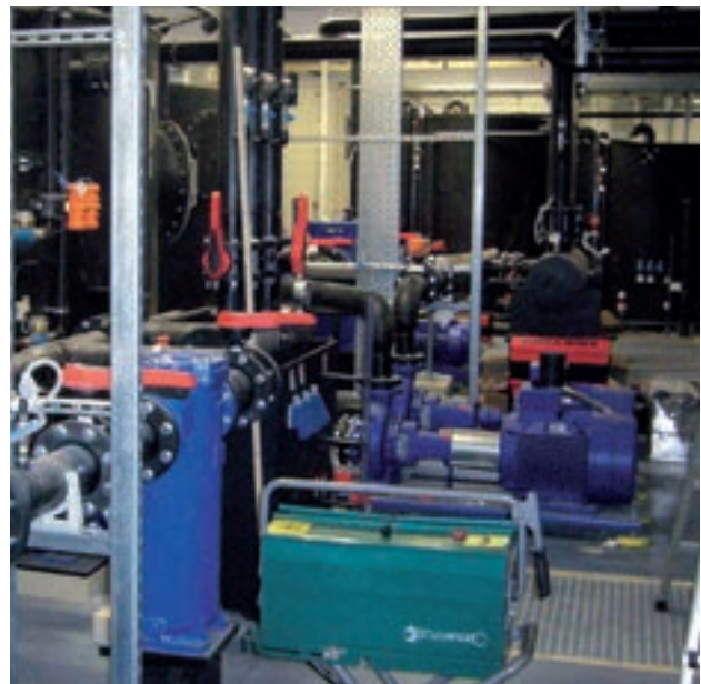
Cooling system for transformers and switch panels.
