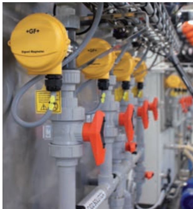
Magmeters ensure high accuracy.
