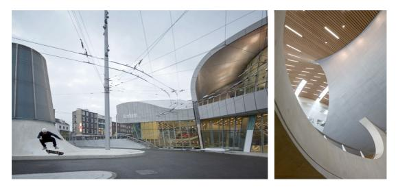
In the development of the design, the practice used a series of conceptual structural tools to mold the geometry of the terminal landscape to accommodate the different programme functions. These include the use of 'V-walls', a load-bearing concrete structure that absorbs the differences in the required grids and provides daylight to the below ground levels. The spaces between these elements also form the public access from the underground car park to the other components.
